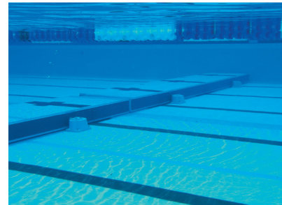
Bulkhead flat against pool floor
