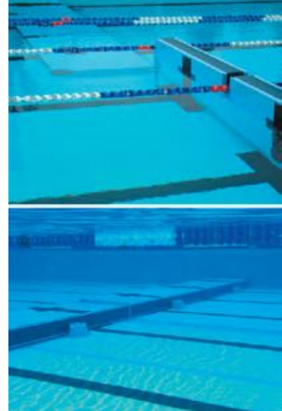
Bulkhead flat against pool floor
